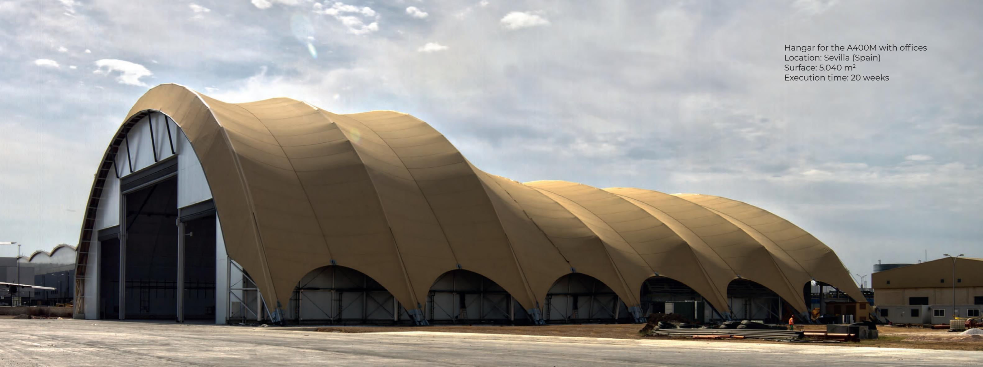
**The structures are composed of structural aluminium profiles with mechanical joints.**
